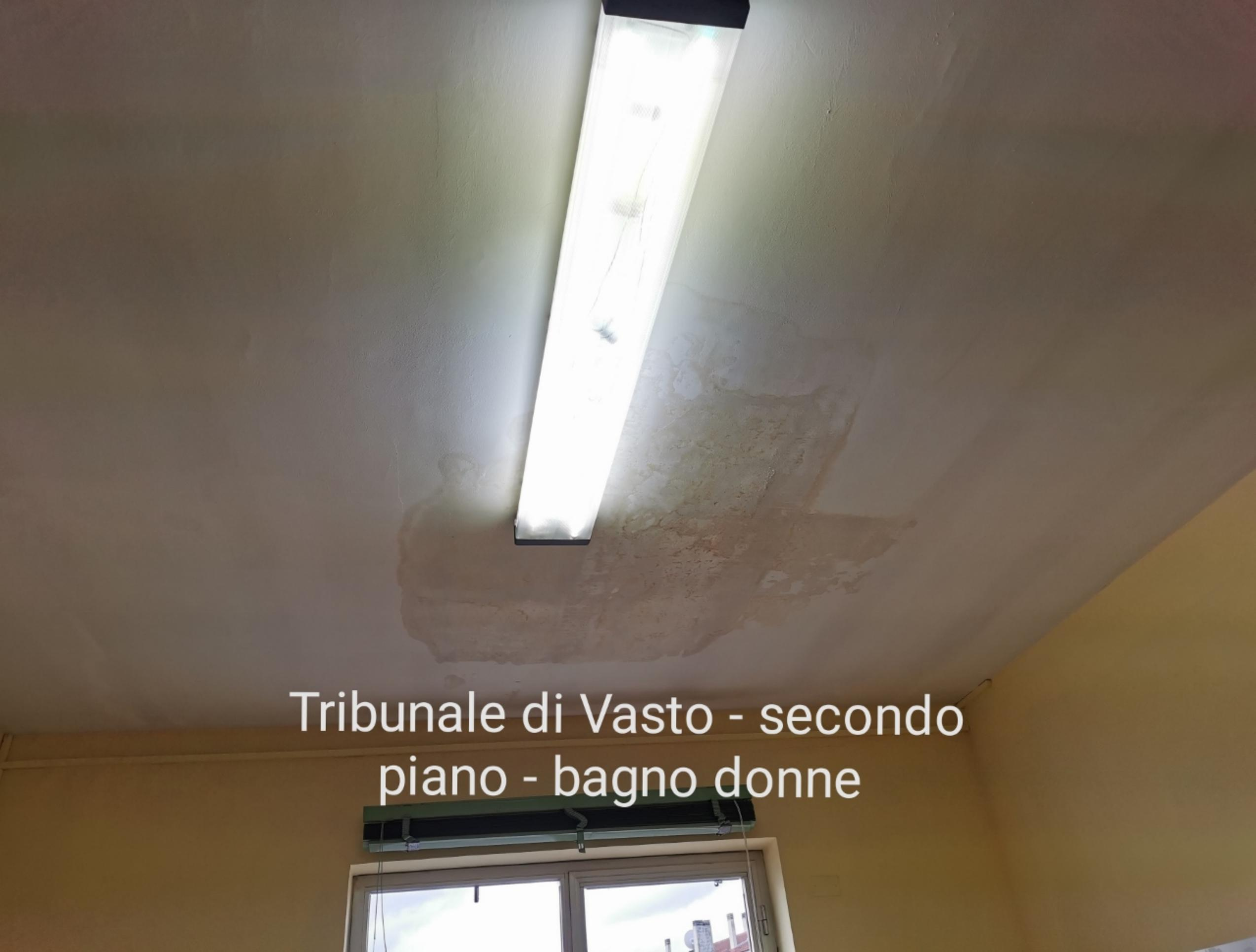
A photograph of a ceiling in a bathroom. A large, irregular, brownish water stain is visible on the white ceiling, centered around a rectangular fluorescent light fixture. The stain has a darker, more saturated center and fades out towards the edges. The light fixture is illuminated, casting a bright glow. Below the ceiling, a window with a dark frame and a black roller blind is visible. The wall to the right is painted a light yellow color.
