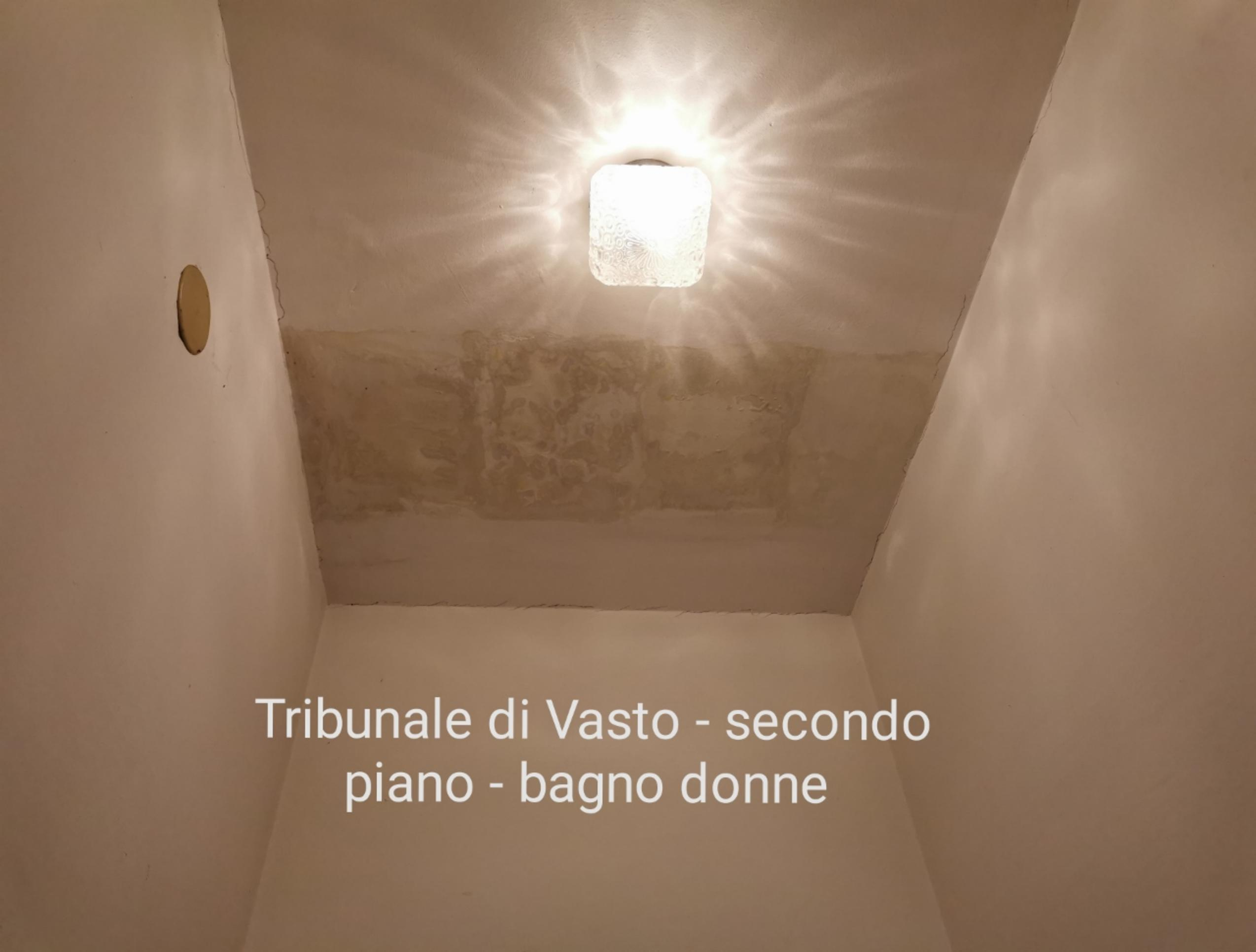
A photograph of a bathroom ceiling. In the center, there is a square, recessed light fixture with a textured, frosted glass cover. The light is on, casting a warm glow. Below the light fixture, there is a large, irregular, brownish water stain on the ceiling. The ceiling is otherwise plain and light-colored. On the left side, there is a small, oval-shaped hole in the wall. The overall scene suggests a plumbing issue in a public restroom.
